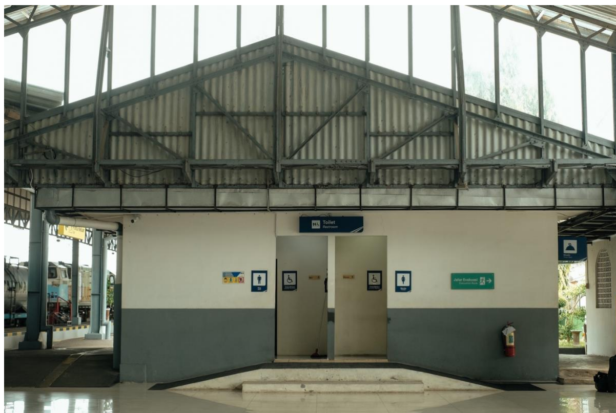
An example of accessible design in Solo. The gradient and material selection for the ramp is not ideal.
