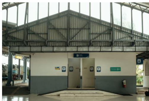
An accessible bathroom in a train station in Solo.
