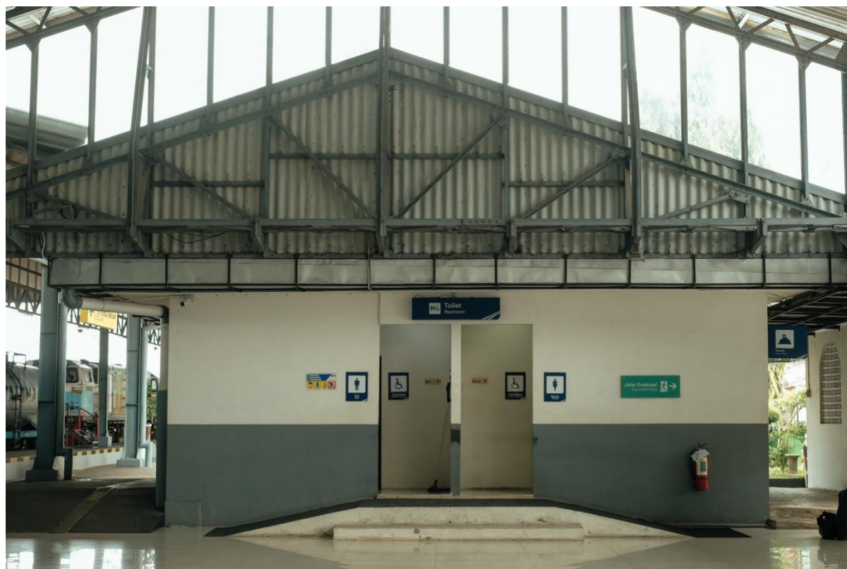
An example of accessible toilets in a train station in Solo.
