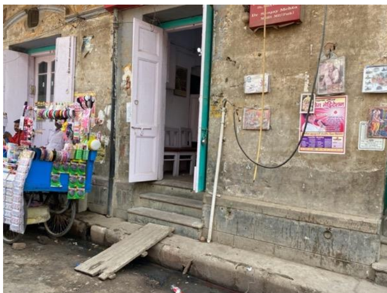
Existing building stock must be made accessible.
