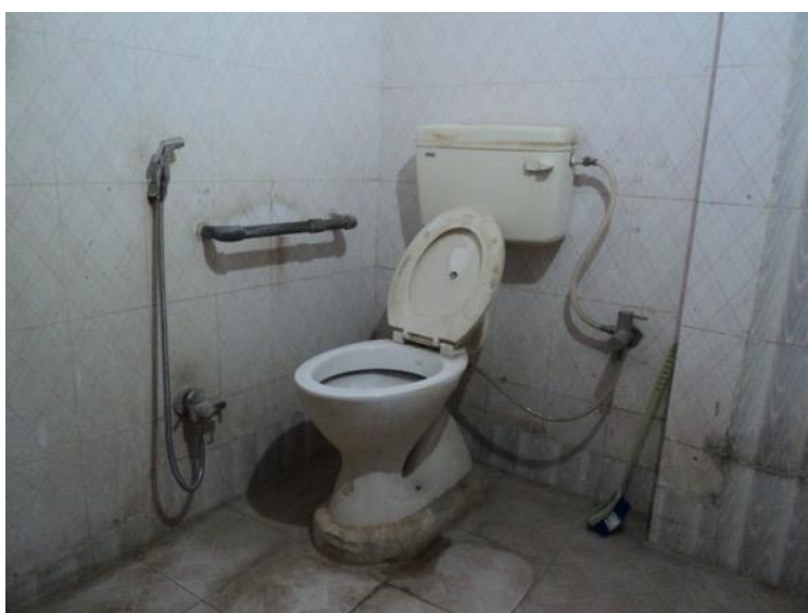
An example of an accessible toilet that has not been well maintained.
