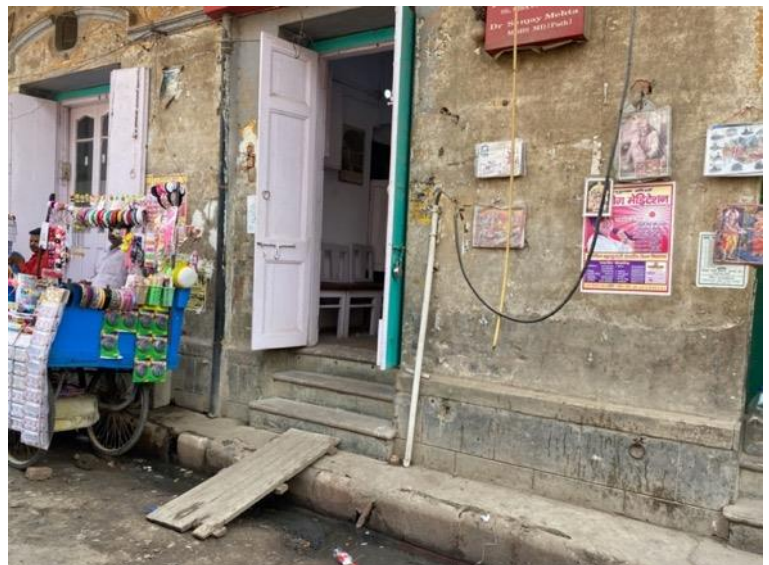
Existing building stock must be made accessible.
