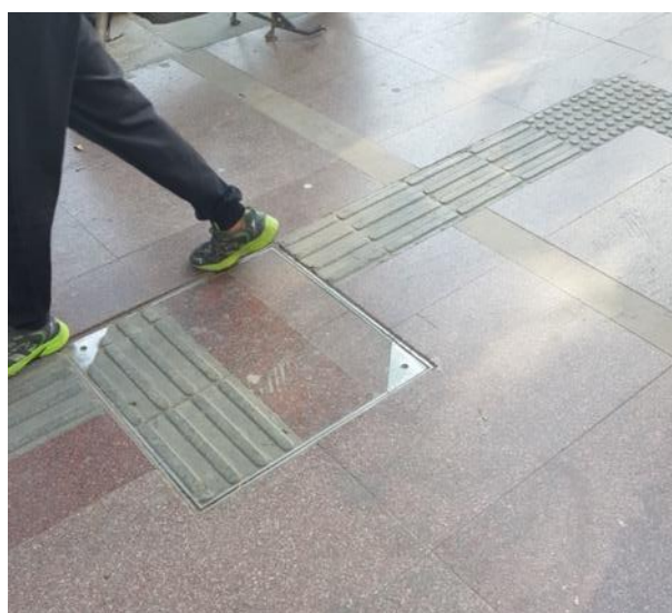
This photograph of tactile paving in Delhi illustrates the importance of good maintenance of inclusive environments.
