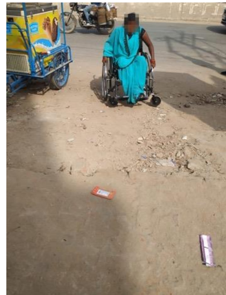
Poor road conditions and a lack of pedestrian infrastructure.
