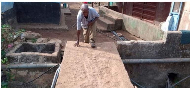
Example of bridge over drain
