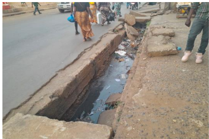
Example of open drainage on streets
