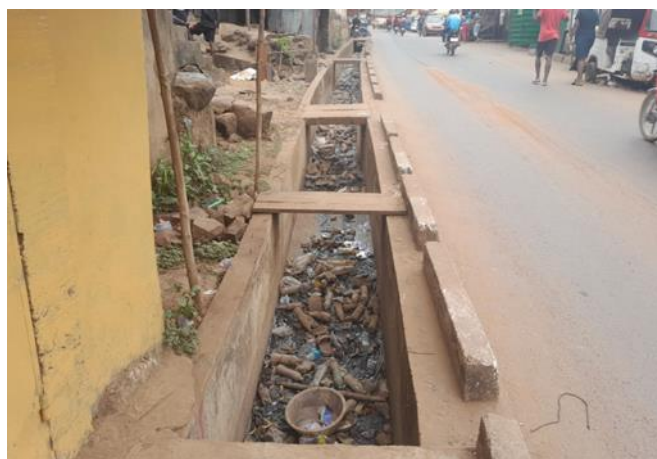
Example of open drainage on streets
