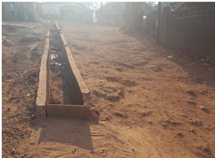
Informal drainage system
