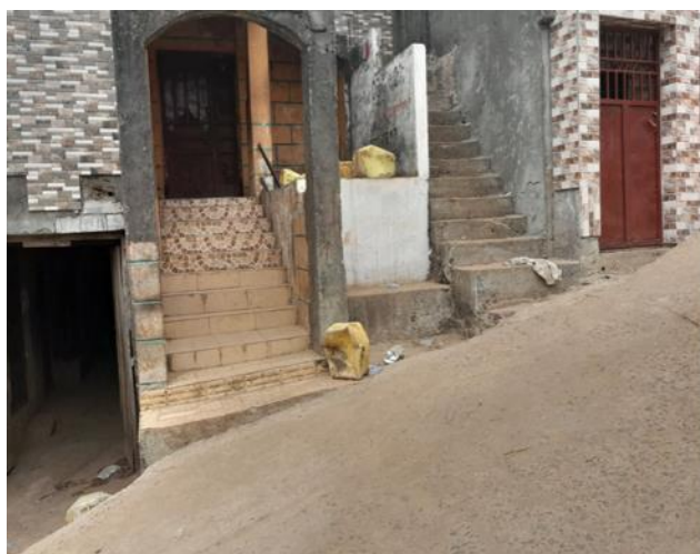
An example of inaccessible steps leading to housing
