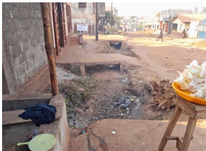
Example of a ramp into a home over a drain
