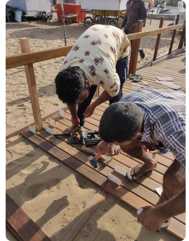
Two men using a hammer and a drilling machine to fix the timber planks of the access ramp to the beach.
